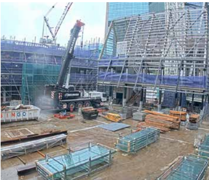
The Plaza Building and plaza construction progress in March 2022
