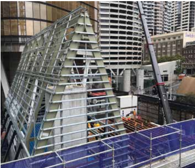
The Plaza Building taking shape in March 2022
