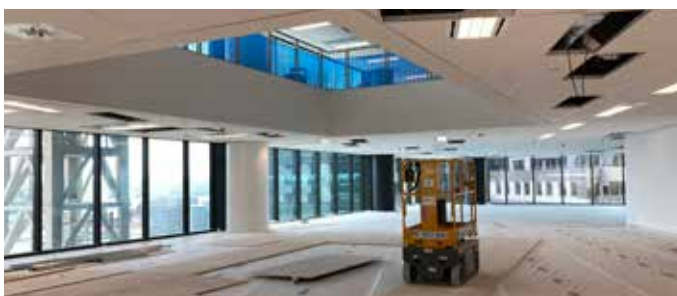
Left: Finishes work on Level 6
